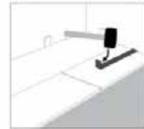
8. Use mallet & pull bar to lock in final board in row. Insert spacer between end of row and wall to ensure flooring maintains position through full install process.
